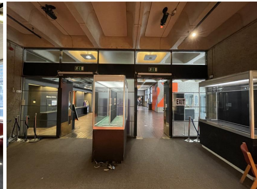
View from Library foyer toward lift lobby. Door D01 to be formed in right hand panel.
