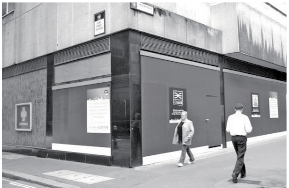
Crossrail hoardings on the former Boots at the corner of Moorfields and Fore Street Avenue
