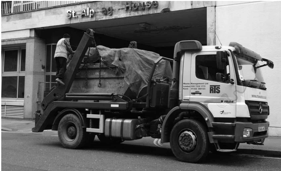
The demolition of St Alphe House is to start shortly
